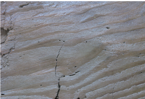
2. Cavities, damaged surfaces (Anjwado shipwreck)
