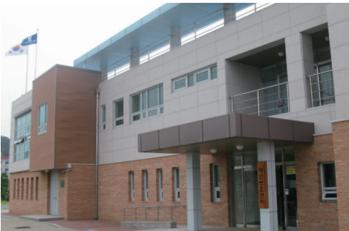
2. Taeon conservation centre
